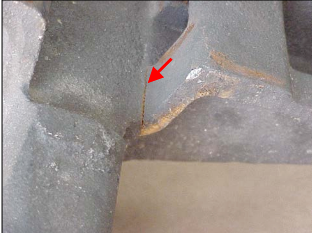
Photo 3: Submitted Sample #2, cracking at arrow.
